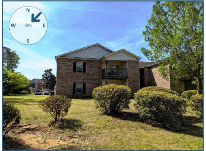
View of site from the northeast
