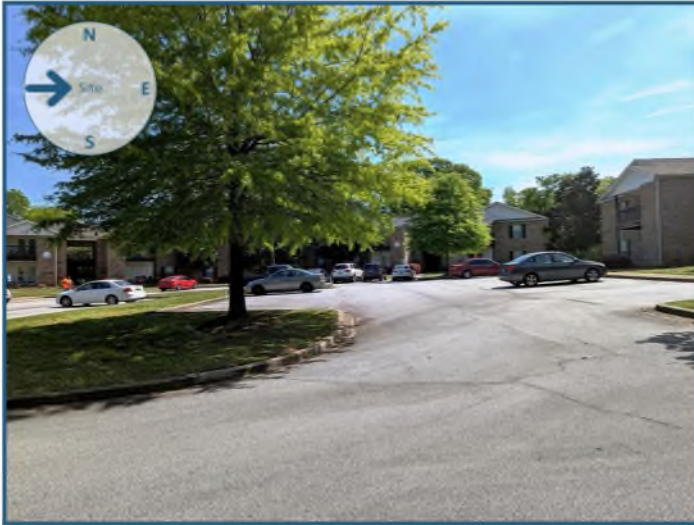
View of site from the west
