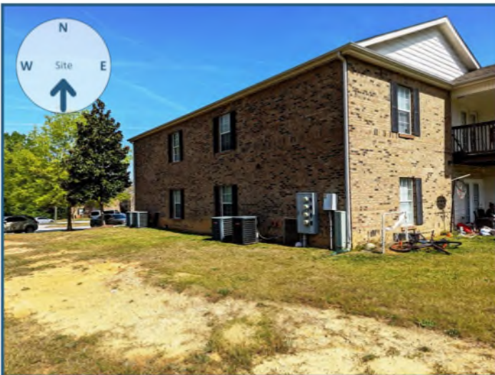
View of site from the south
