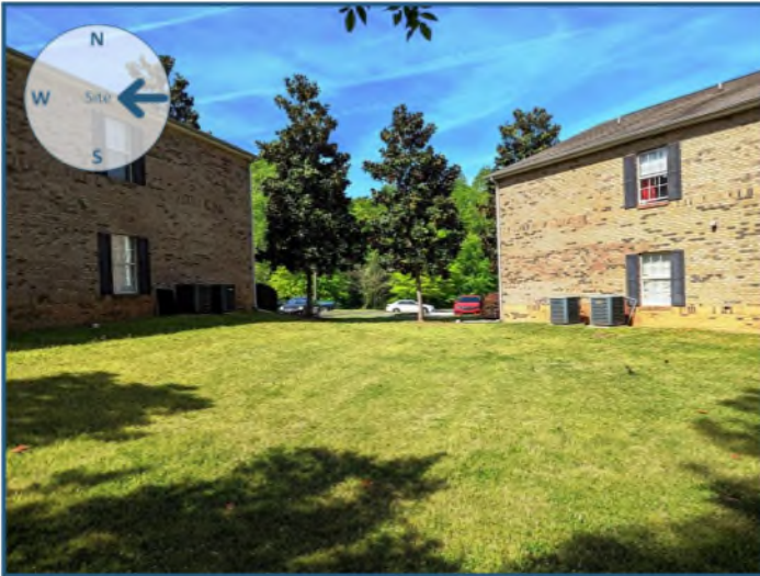
View of site from the east
