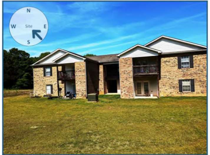
View of site from the southeast
